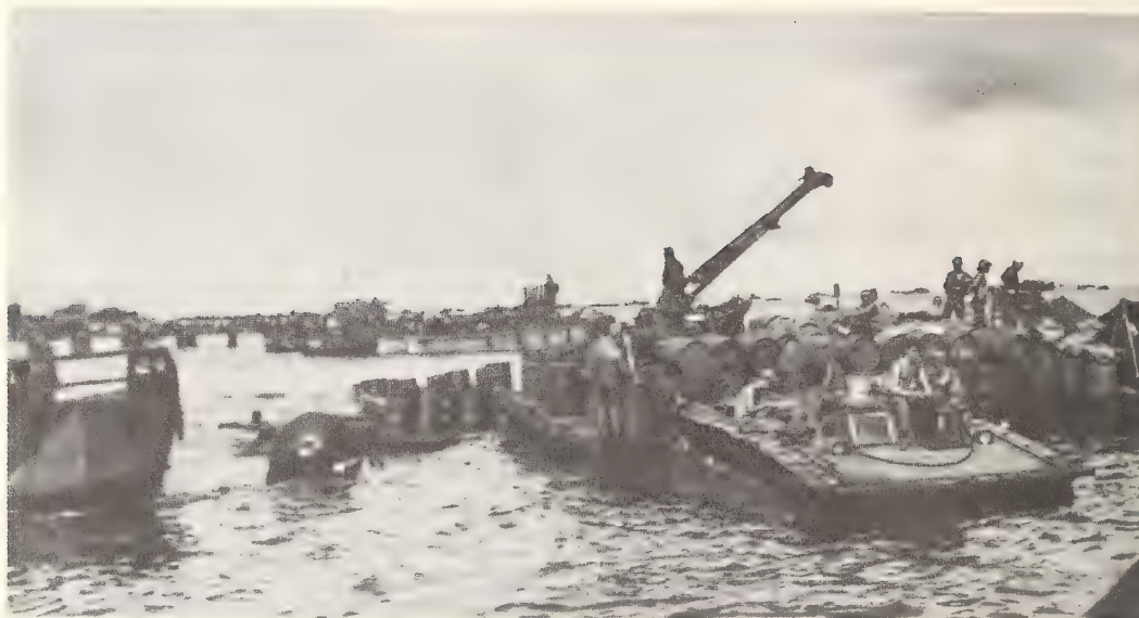
PONTOON BARGE loaded with fuel drums at the reef transfer line off Guam. (USA SC210553)
